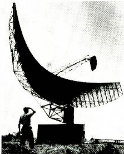
Five-ton radar antenna is 41 feet wide.
